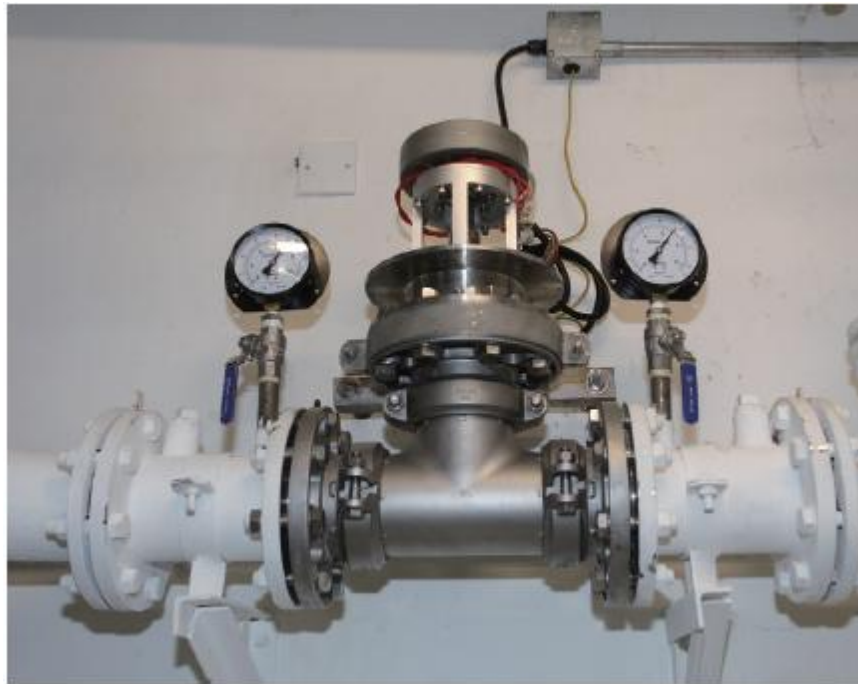
Figure 5: The Compact Turbine for Generation of Hydro Power at Olympian City 2
